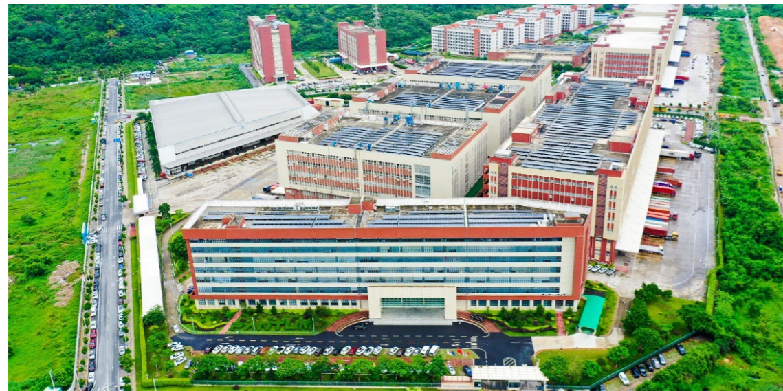
Photovoltaic power generation equipment on the roof of factory buildings
